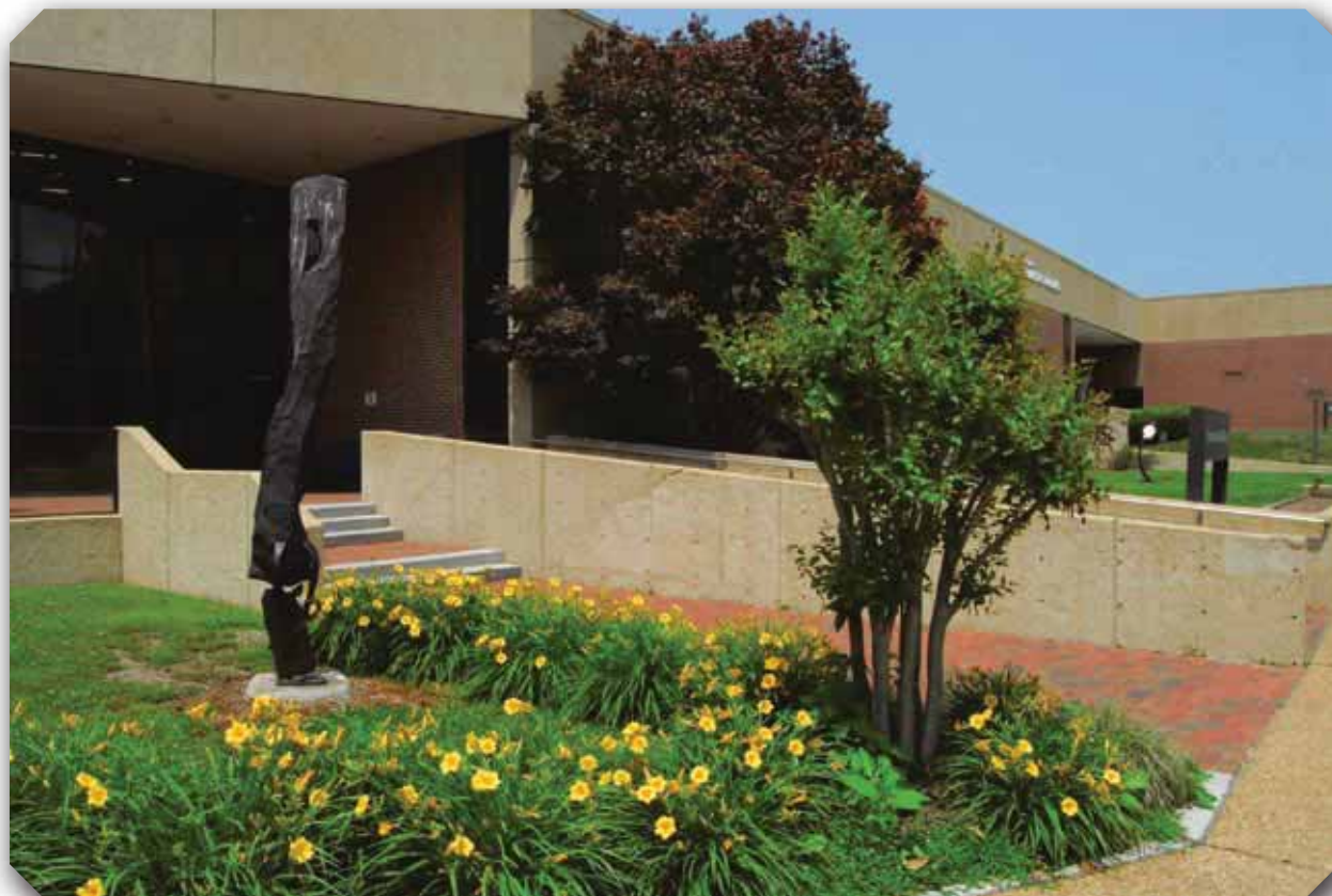
Chattanooga State's C.C. Bond Humanities building contains an auditorium, class rooms, labs and offices.
